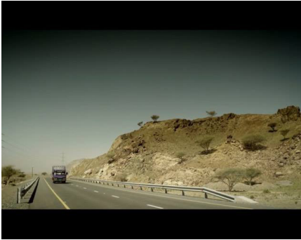
Figure 3: the concrete road
